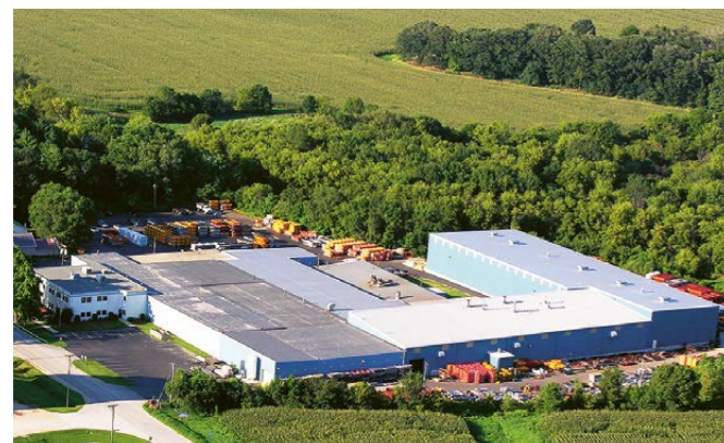
Cleveland and Lindenwood, USA
